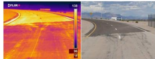
Thermal infrared (left) and visible (right) images of a road with light and dark segments. The infrared image shows that the light segment (bottom) is about 17°C (30°F) cooler than the dark segment (top). (Image courtesy of Larry Scofield, APCA)
