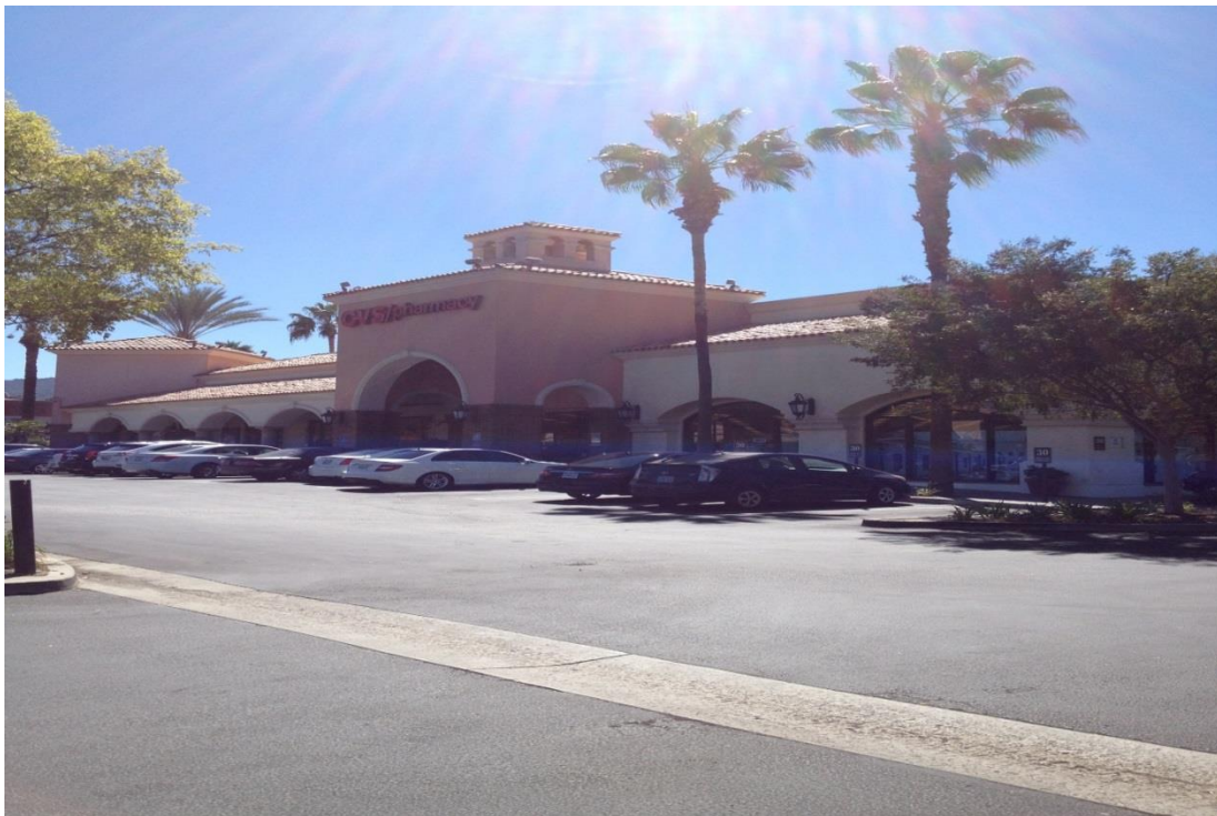
8. 16461 Ventura Blvd: looking south west at the east side entrance.
