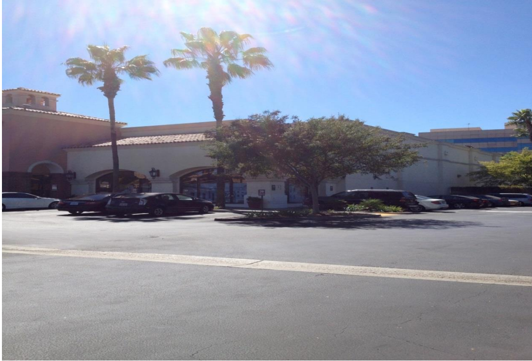
7. 16461 Ventura Blvd: facing north west from the west corner parking lot of the subject property.
