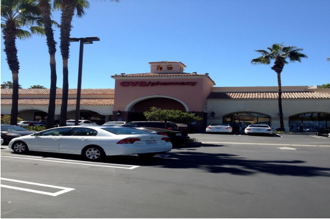
1. 16461 Ventura Blvd: looking west at the east side entrance of the subject property.
