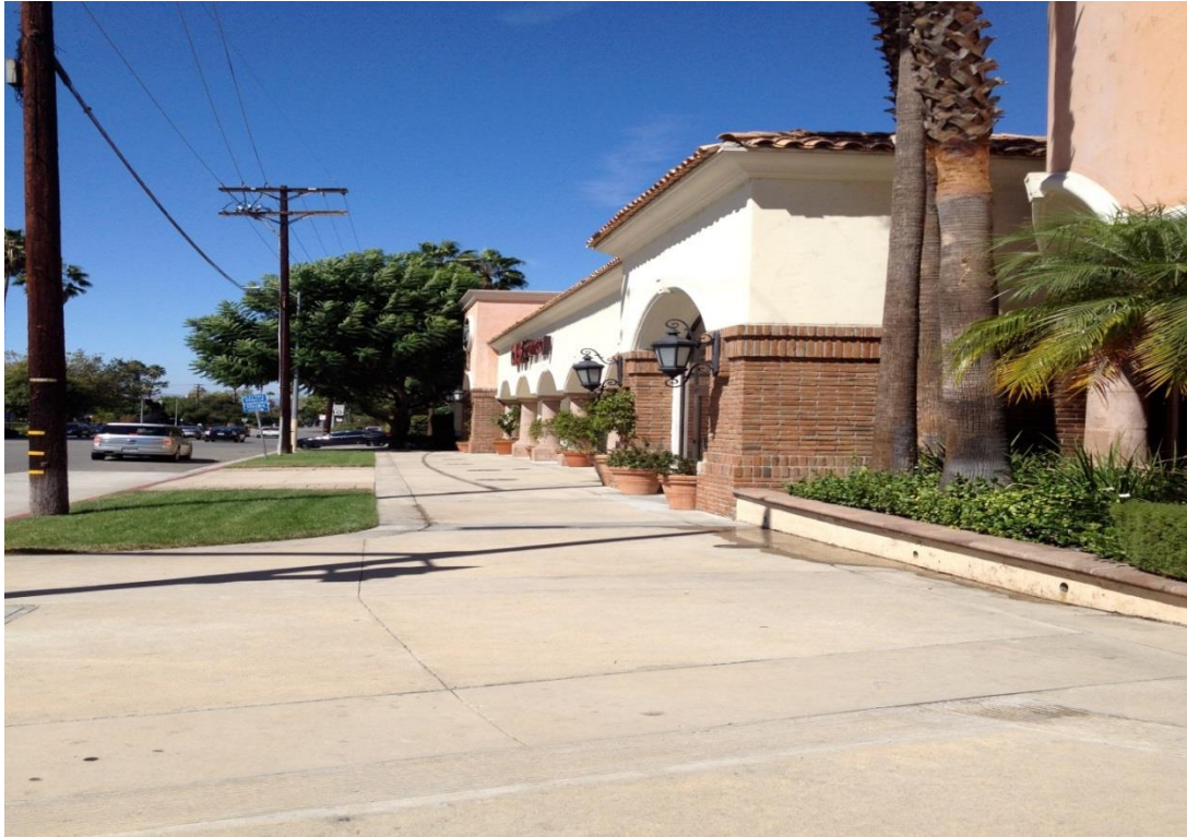
22. 16461 Ventura Blvd: facing north from the west side of the subject property.
