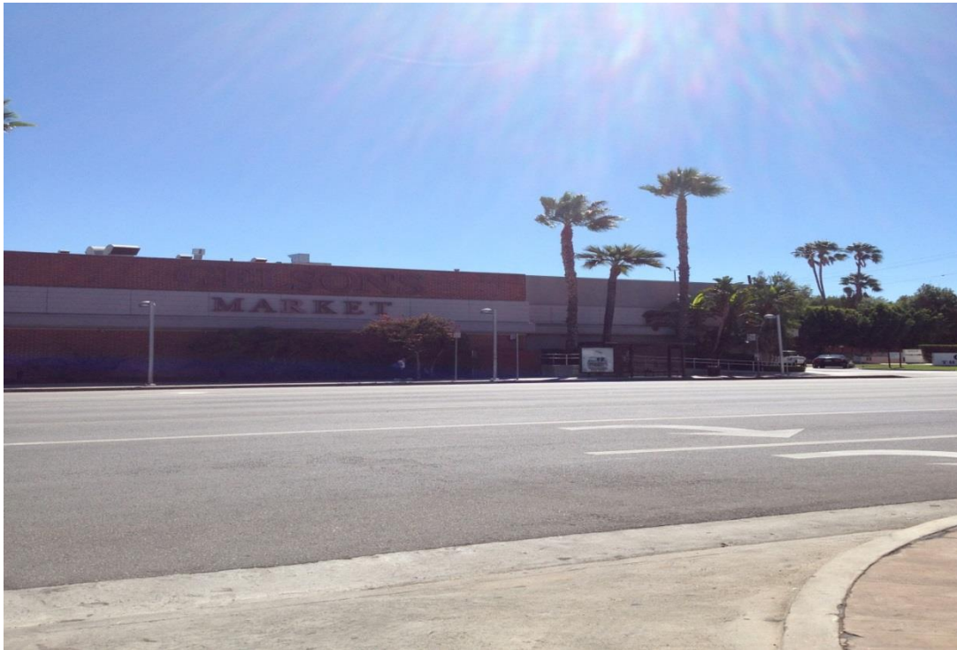
12. 16461 Ventura Blvd: facing south west from the south east entrance of the subject property.
