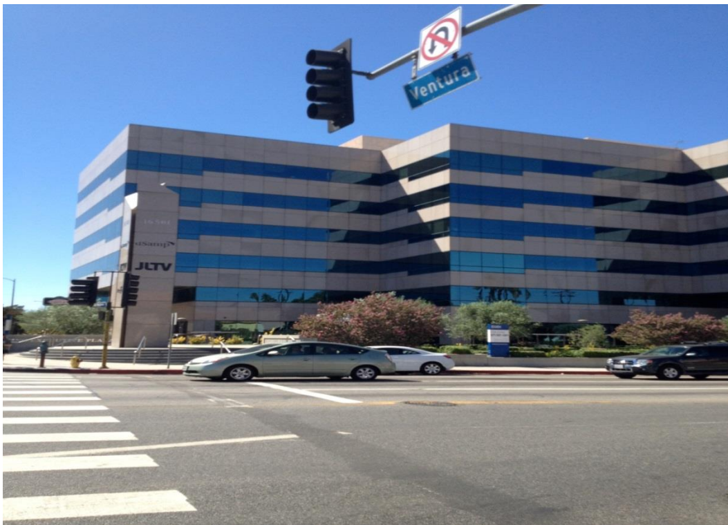
24. 16461 Ventura Blvd: facing west from the south west corner of the subject property.
