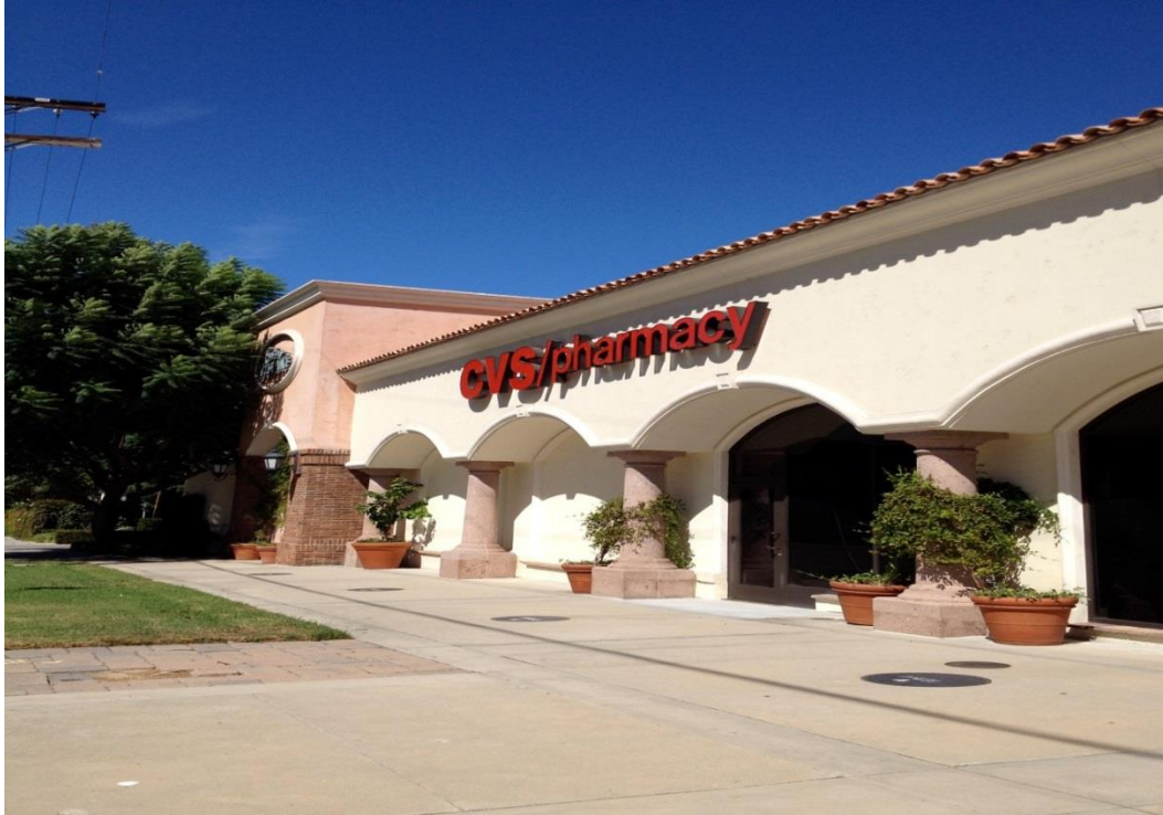
27. 16461 Ventura Blvd: facing north from the west side of the subject property.
