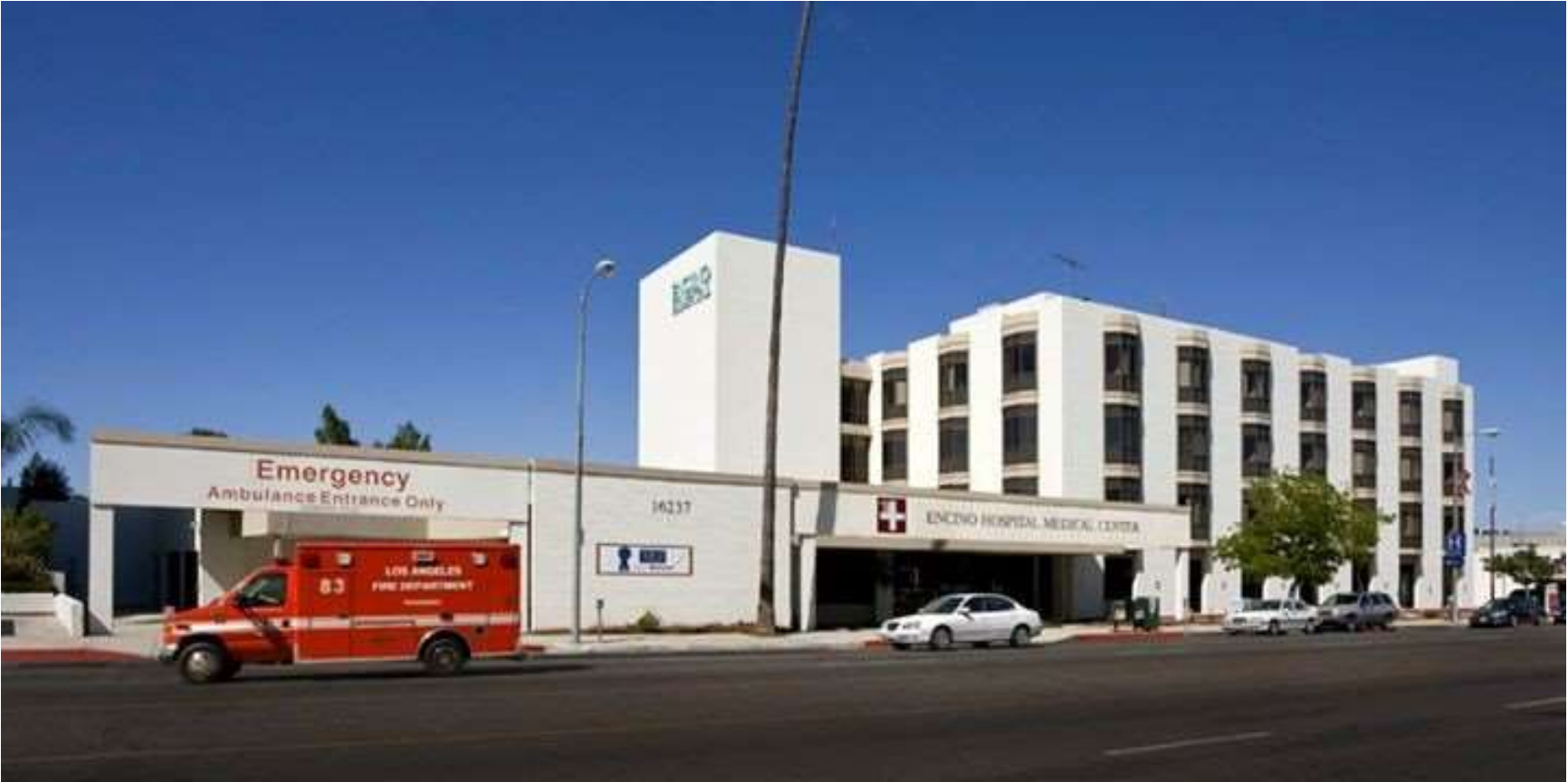
Photo 1: View of Hospital along W. Ventura Boulevard
